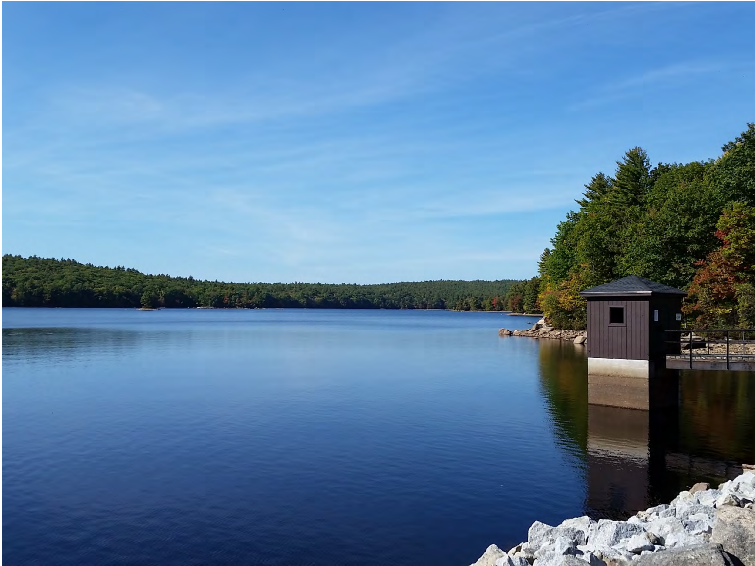
Tower Hill Pond Project 1800 + Acres
